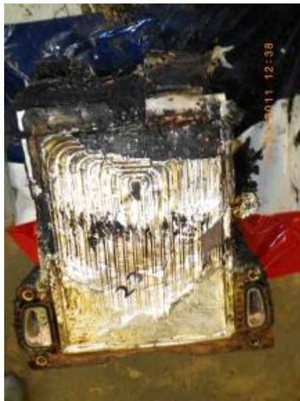
Figure 7.9 – Photograph Showing Cell Level Damage within Module 3
