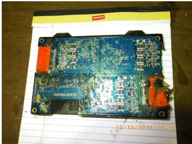
Figure 7.16 – VTSM 3 – No Apparent Fire Damage
